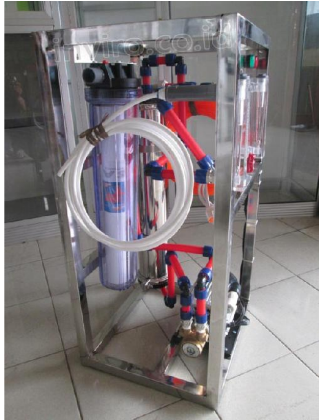
Gambar item no. 1 diatas, Unit Rangkaian Mesin RO (Reverse Osmosis) 1.000 GPD Vontron/setara (Setara 200 Galon/Hari, 1 Galon = 19 Liter)
